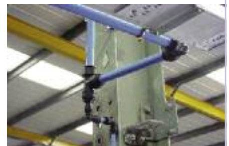
5. System complete in 2 days
